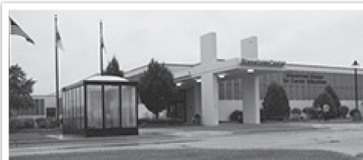
Stenstrom Center for Career Education (SCCE), formerly Samuelson Road Center (SAML) located at 4151 Samuelson Road, Rockford, IL 61109 just east of Rockford Jefferson High School
