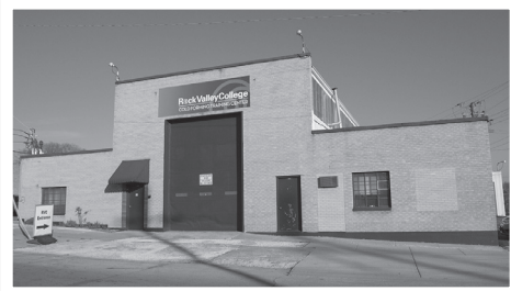
Cold Forming Training Center (CFTC) located at 424 Buckbee Street Rockford, IL 61104;
